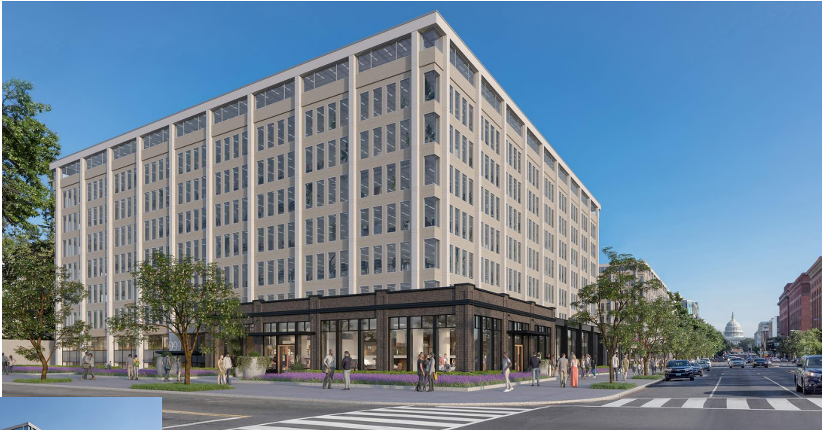
999 N Capitol - Looking Southeast
