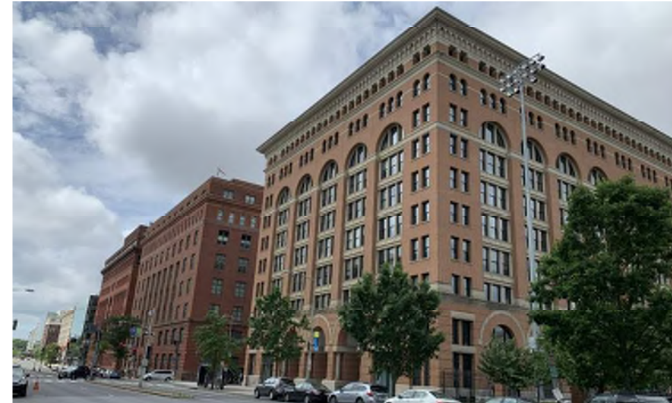
4 ACROSS NORTH CAPITOL STREET - VIEW LOOKING SOUTHWEST
